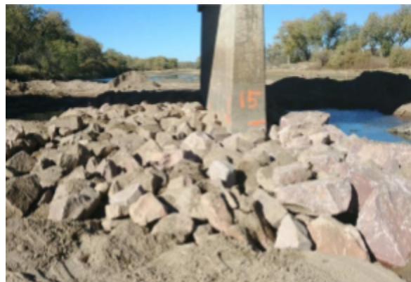
Photo 17.2 Rock riprap installed as pier-scour countermeasures at US 6 in the South Platte River near Merino, Colorado.
