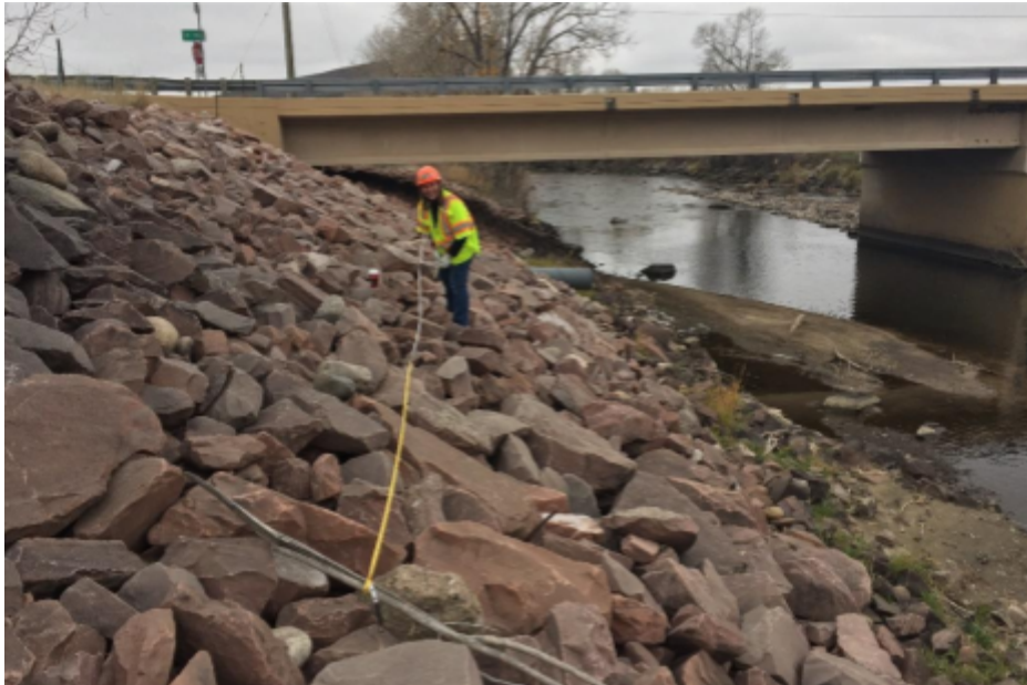
Photo 17.5. Collecting Wolman Counts of post-construction rock riprap at the Cache la Poudre River adjacent to US 287, Larimer County, Colorado, at MP 355.
