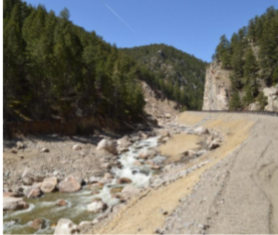
Photo 17.4 The completed matrix-riprap revetment from Photo 17.3 prior to landscaping.
